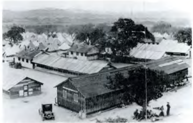
Camp Headquarters Building, 1917. In much-modified form, this building still serves as the camp headquarters.
