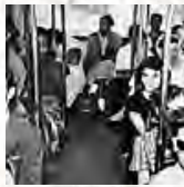
An example of segregation on a city bus
